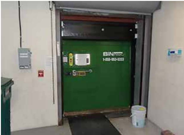
Load BINPAK from inside building
